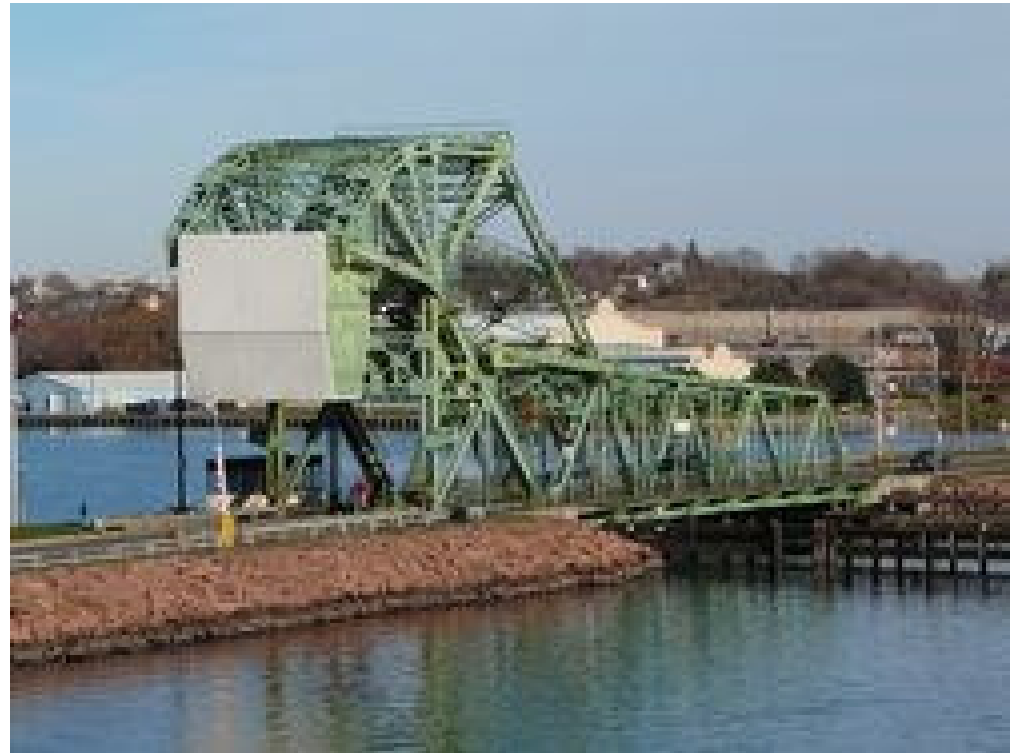
Lasalle Causeway Bridge
