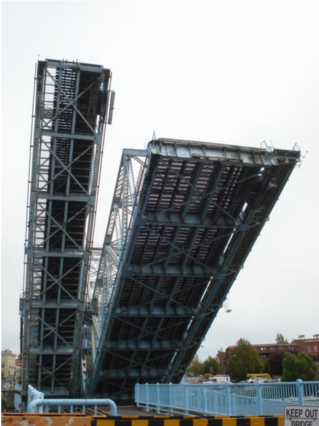
Spans being raised, viewed from the west
