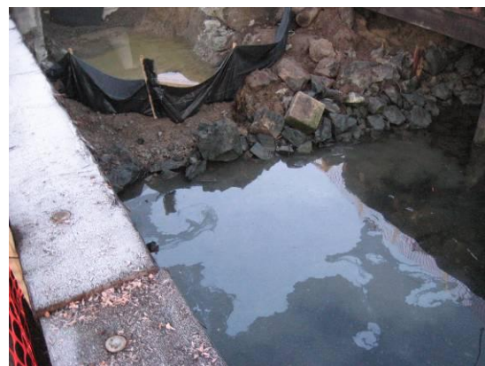
After pile removal – note creosote sheen
