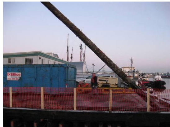
Placing the pile on the adjacent deck
