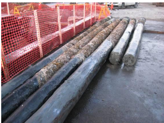
Piles placed on the adjacent deck
